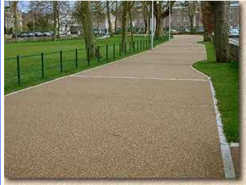
all paths to be resurfaced with new improved drainage
