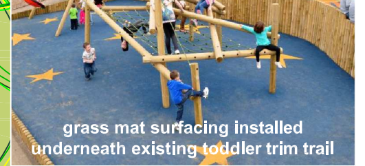
grass mat surfacing installed underneath existing toddler trim trail
