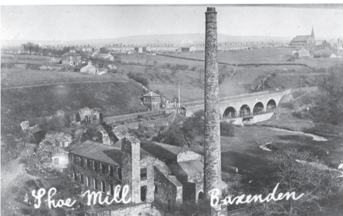
Five Arches Bridge at Shoe Mill
